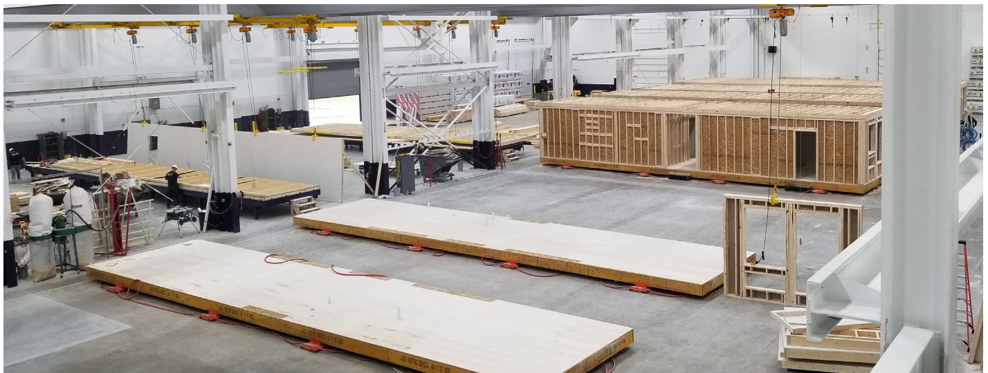
Units on the production floor at the newly-opened Rise Modular factory in Owatonna, MN
